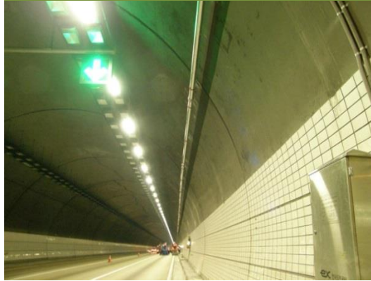
2) Install Main Pipe
