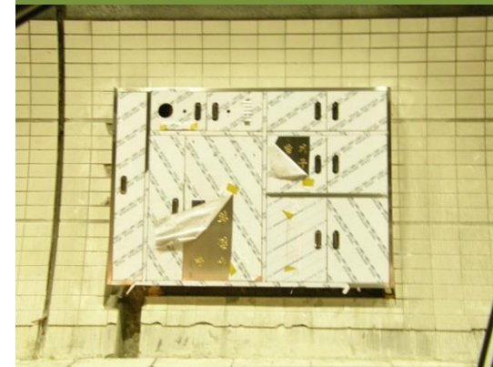
4) Fix Hydrant box
