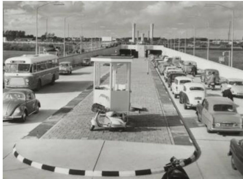
One of the first traffic jams in the history of the country, right after the opening
